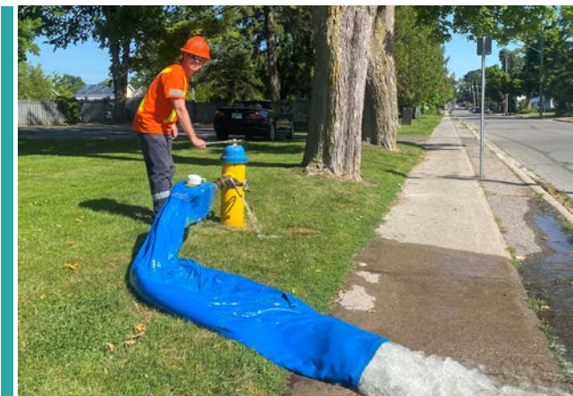
Hydrant Flushing
